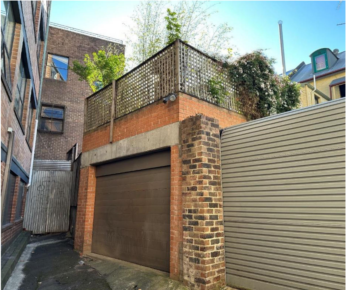
Figure 2. A photo of the raised terrace at the rear of 97 Commonwealth Street. Source: City of Sydney, 2023.
